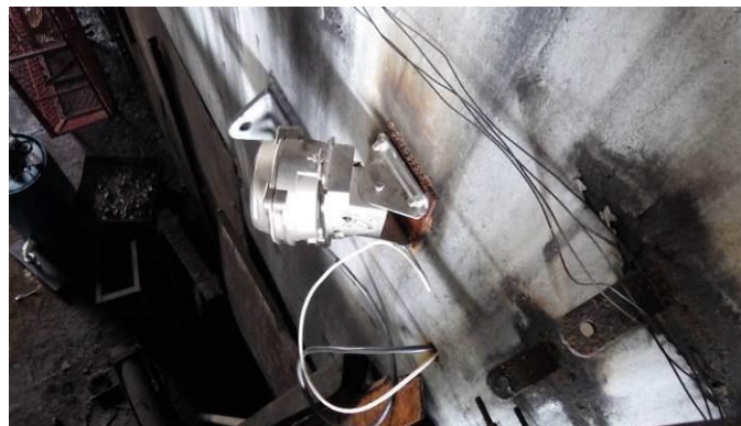
Fig. 12 — Typical Detector Installation (aft/starboard location)
