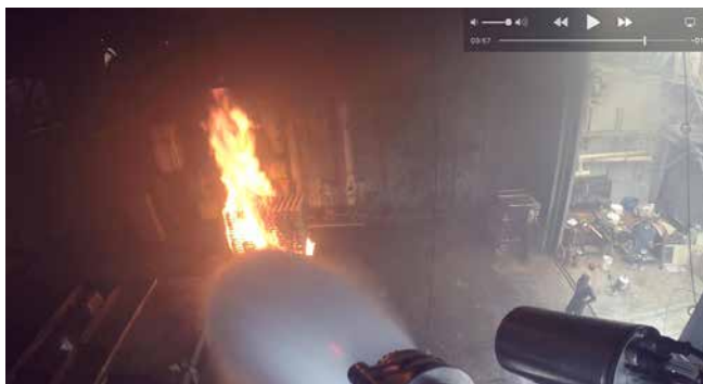
In tests conducted by US Navy, the system have water on the flames within 15 seconds from ignition.
